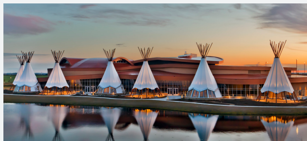
EP provided MEP engineering services for the Shakopee Mdewakanton Sioux Community Hocokata Ti Cultural Center in Shakopee, Minn. It's an example of a project completed with a design-assist approach.
